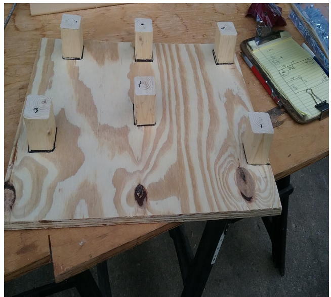
Bottom shelf with blocks in place ready for equipment
