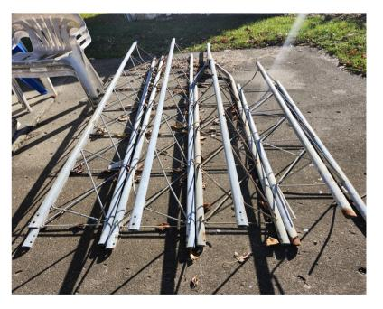
35 foot tubular tower. Has the following sections: 2 - 10 foot, 1 - 9 foot, and 1-6 foot section.
